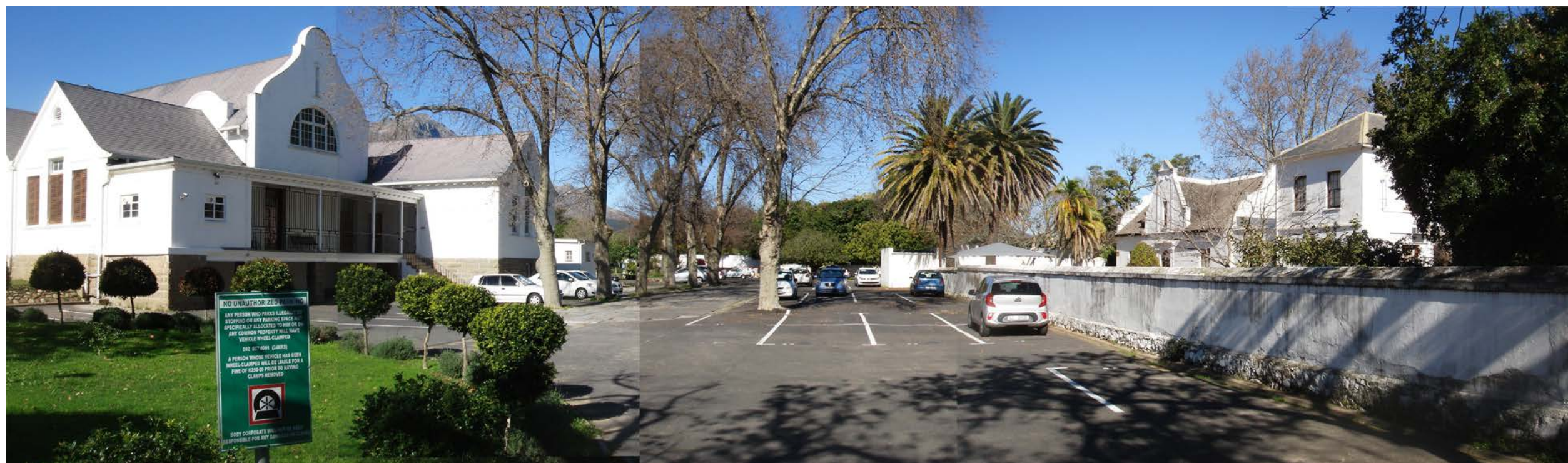
Figure 17: View looking south into area behind the Rhenish School.
