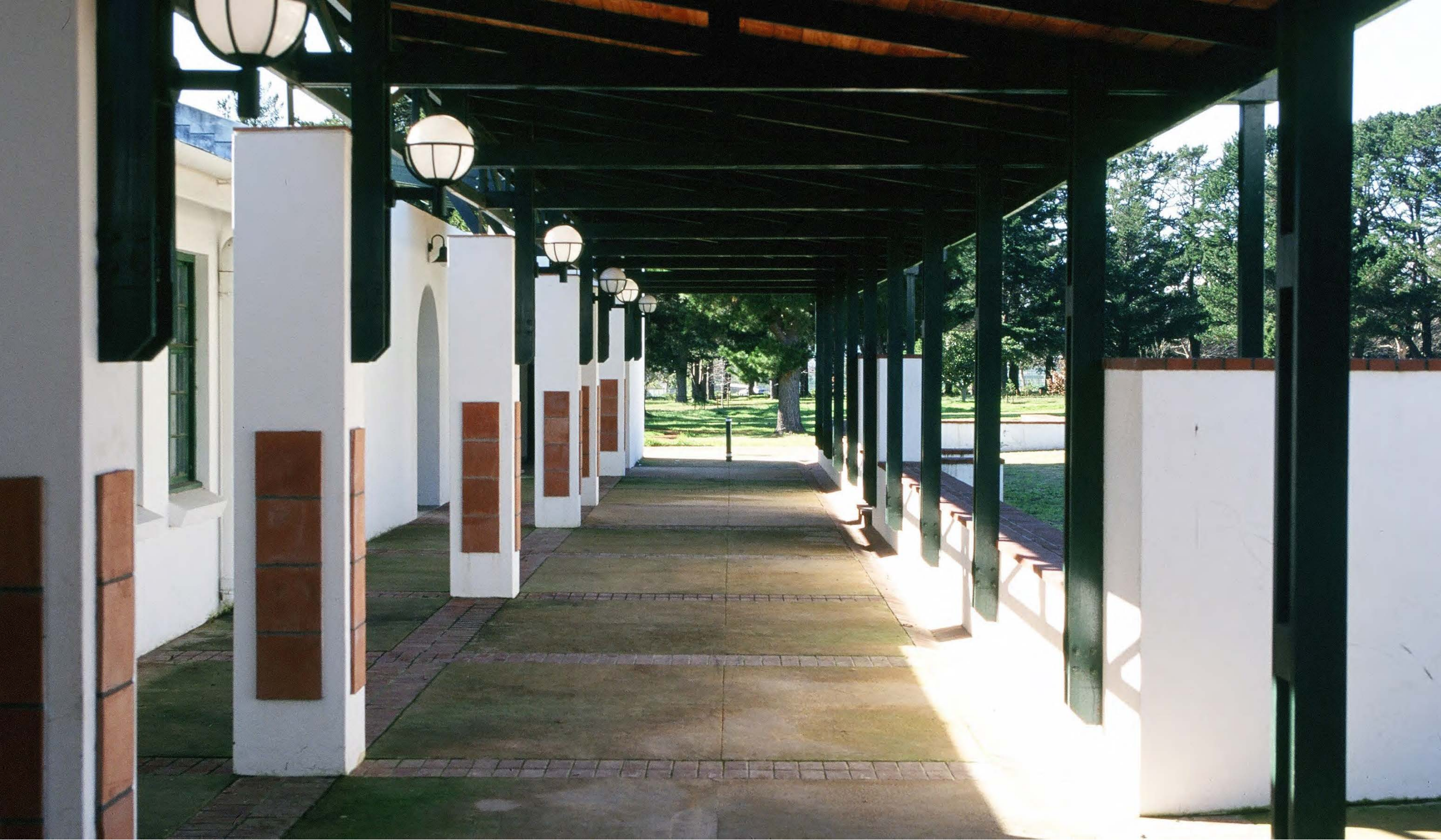
Photograph: Alphen Centre Walkway
