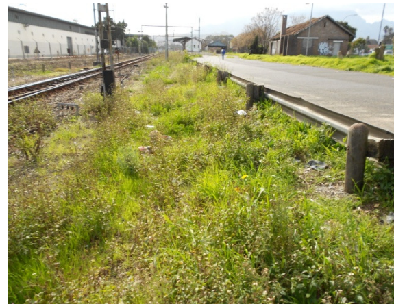
RAIL RESERVE AT STELLENBOSCH STATION
