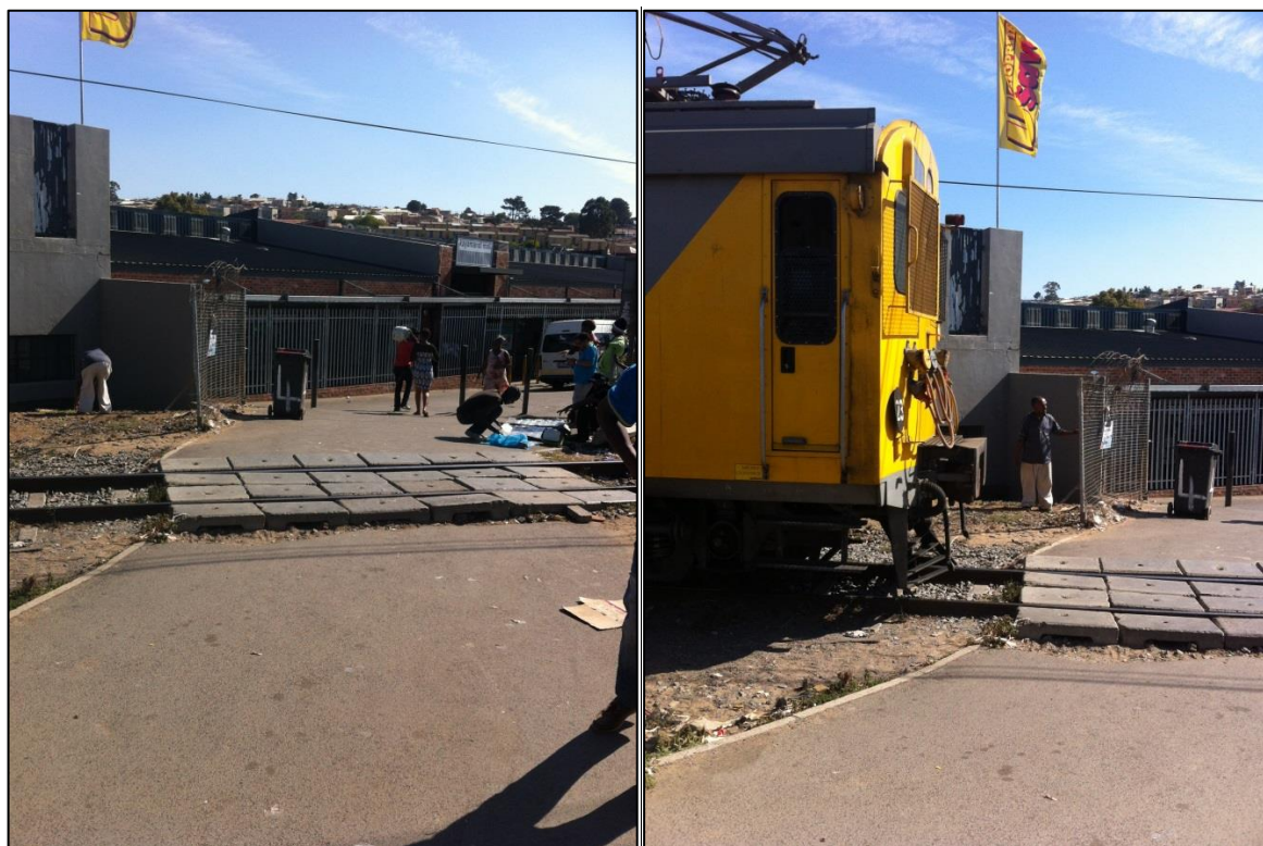
Figure 11-10: Rail Crossing at Kayamandi Mall
