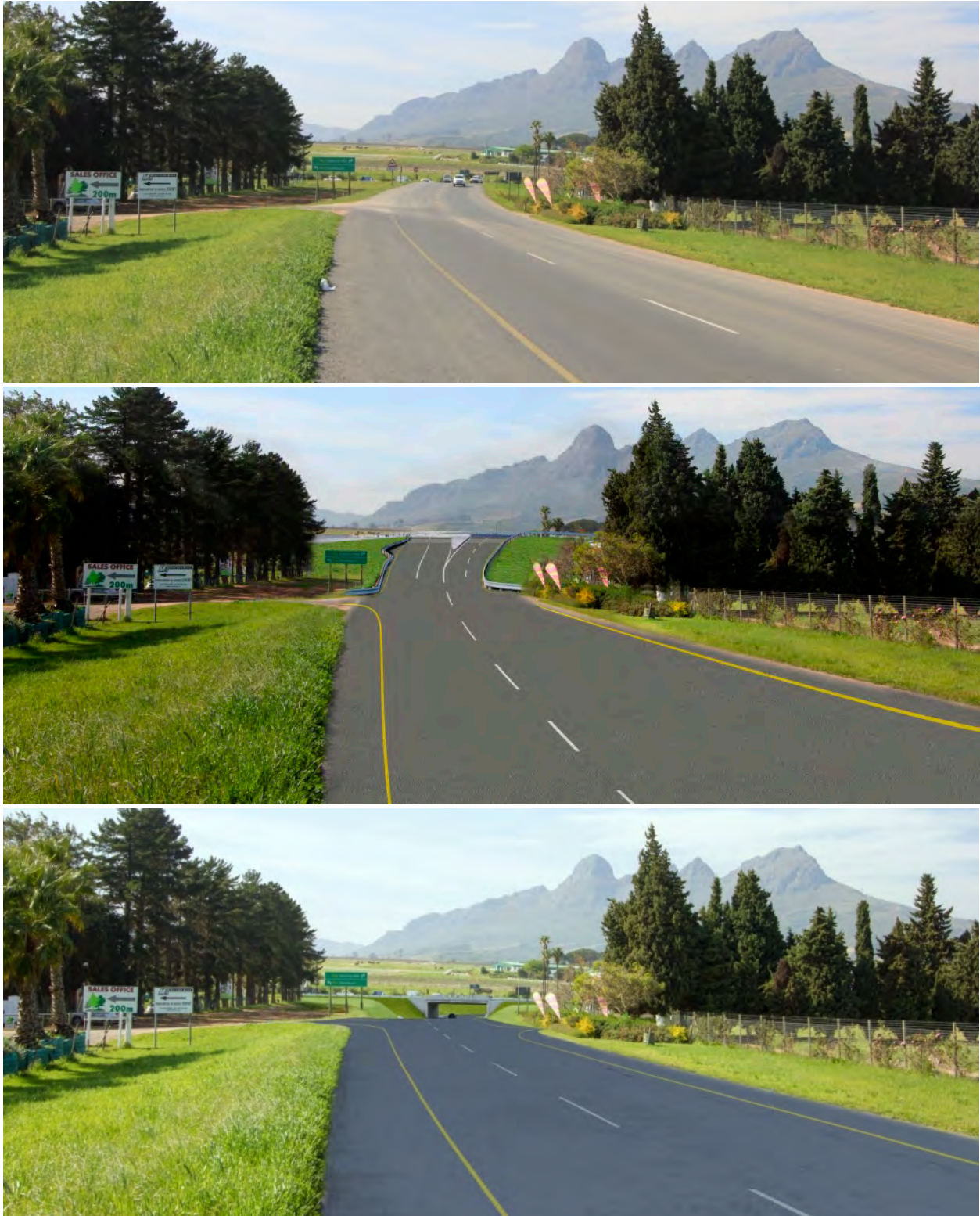
Figure 6.3: Visual simulation of proposed grade-separated alternatives at the R44/Winery Road Intersection, showing the view looking west– composite image comparing an existing view (top image ) with photomontages of the proposed above-ground roundabout (middle image) and the proposed below-ground interchange (bottom image) (Think3dlab, 2016).
