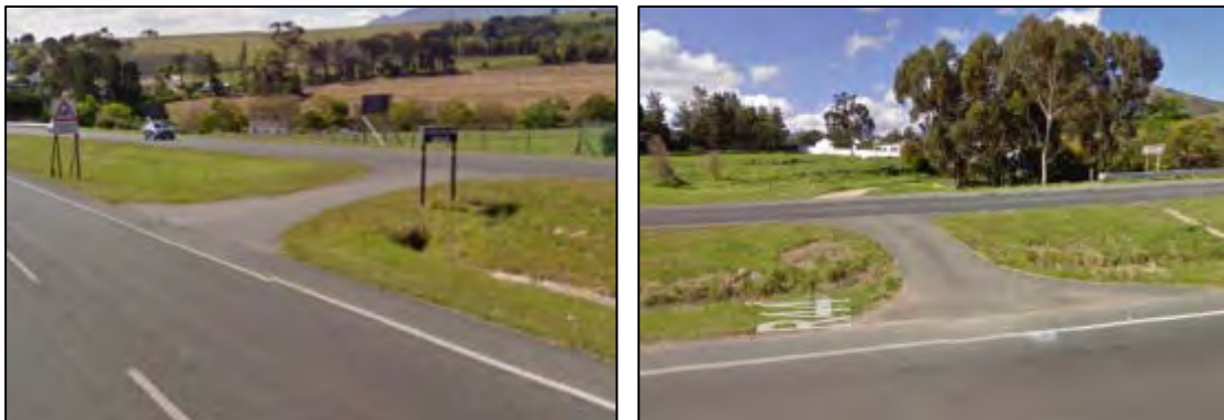
Figure 3.1: Examples of median openings along the R44 (Google street view)
