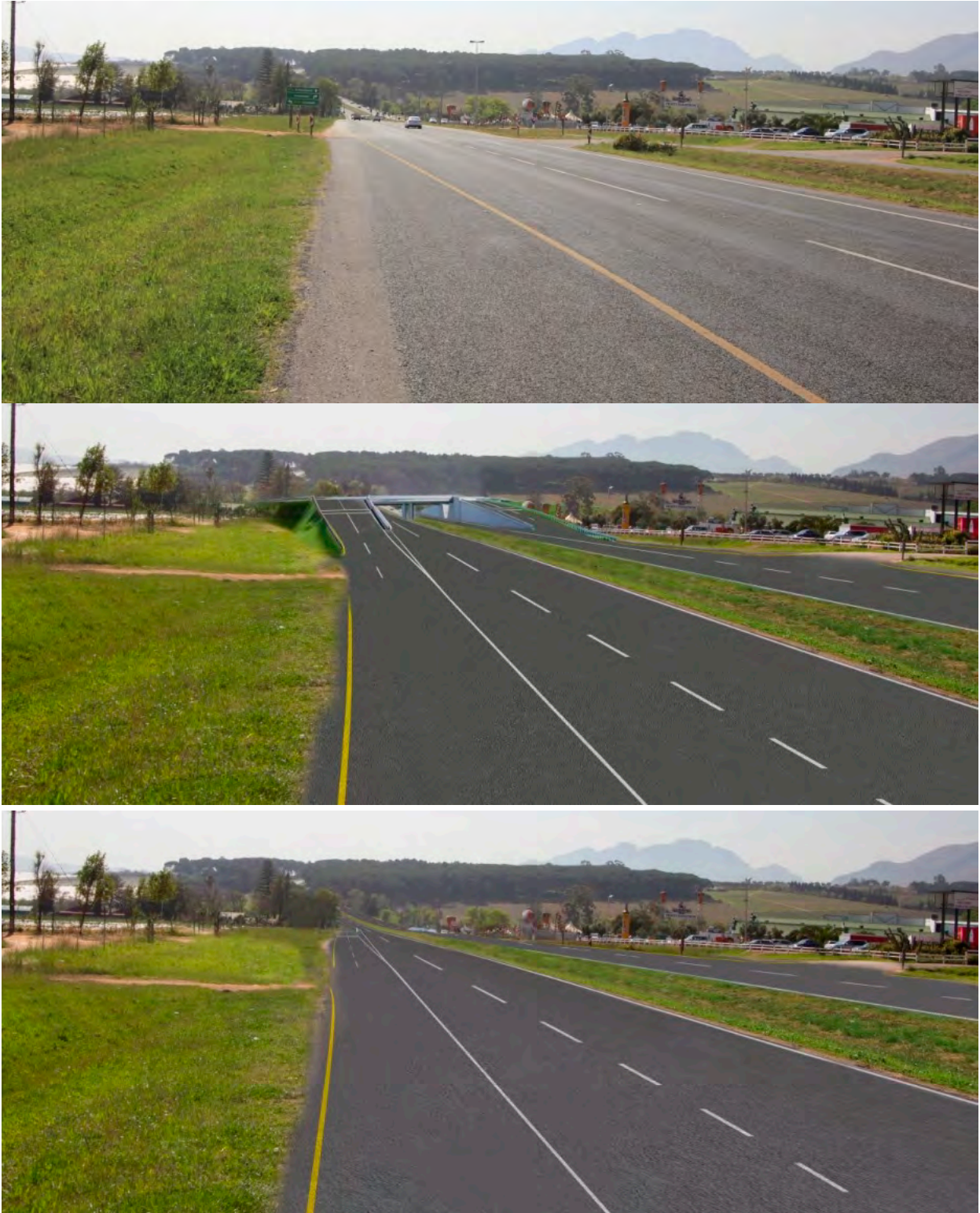
Figure 6.9: Visual simulations of proposed grade-separated alternatives at the R44/Annandale Road Intersection, showing the view looking north – composite image comparing an existing view (top image ) with photomontages of the proposed above-ground roundabout (middle image) and the proposed below-ground interchange (bottom image) (Think3dlab, 2016).
