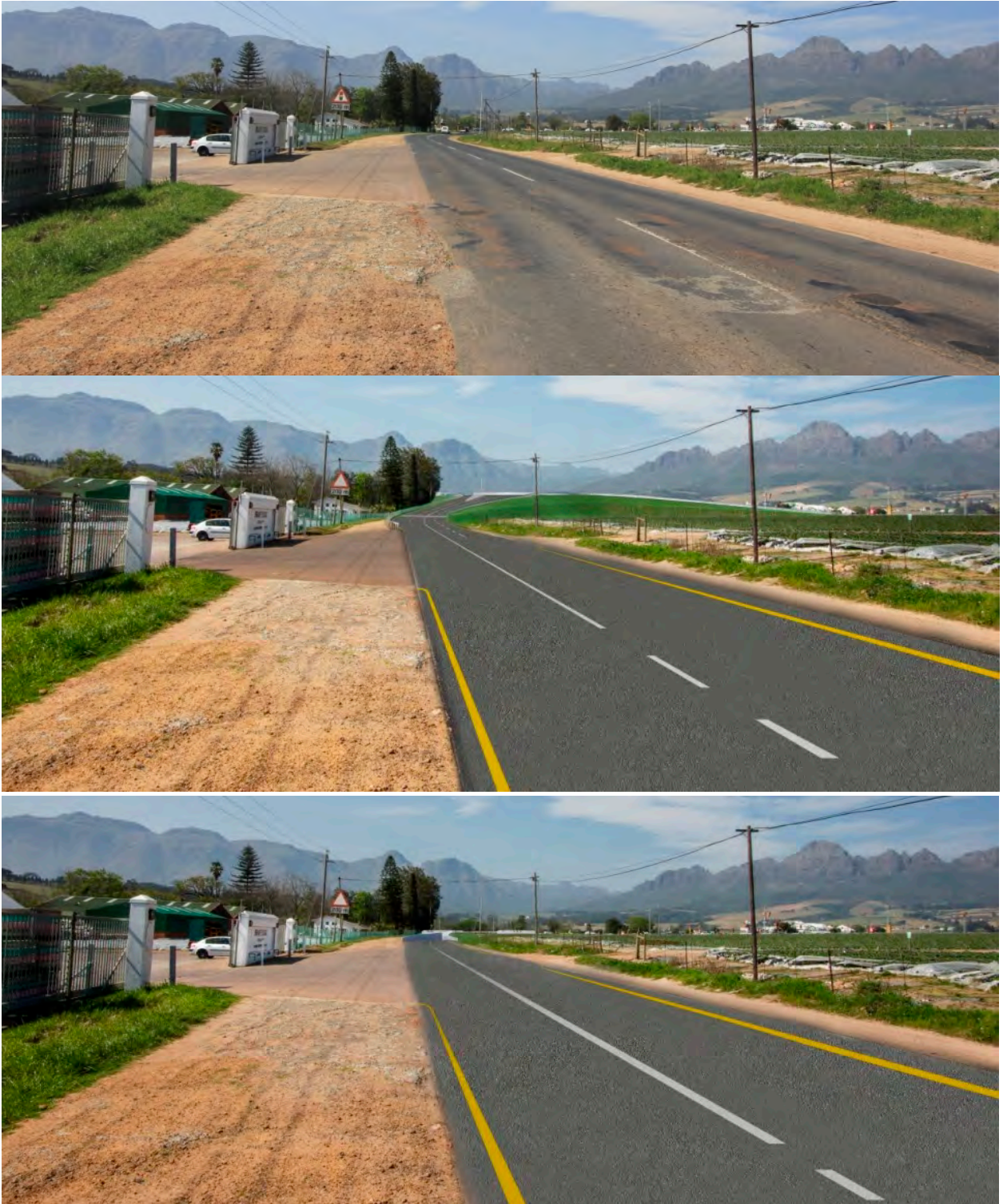
Figure 6.10: Visual simulations of proposed grade-separated alternatives at the R44/Annandale Road Intersection, showing the view looking west – composite image comparing an existing view (top image ) with photomontages of the proposed above-ground roundabout (middle image) and the proposed below-ground interchange (bottom image) (Think3dlab, 2016).
