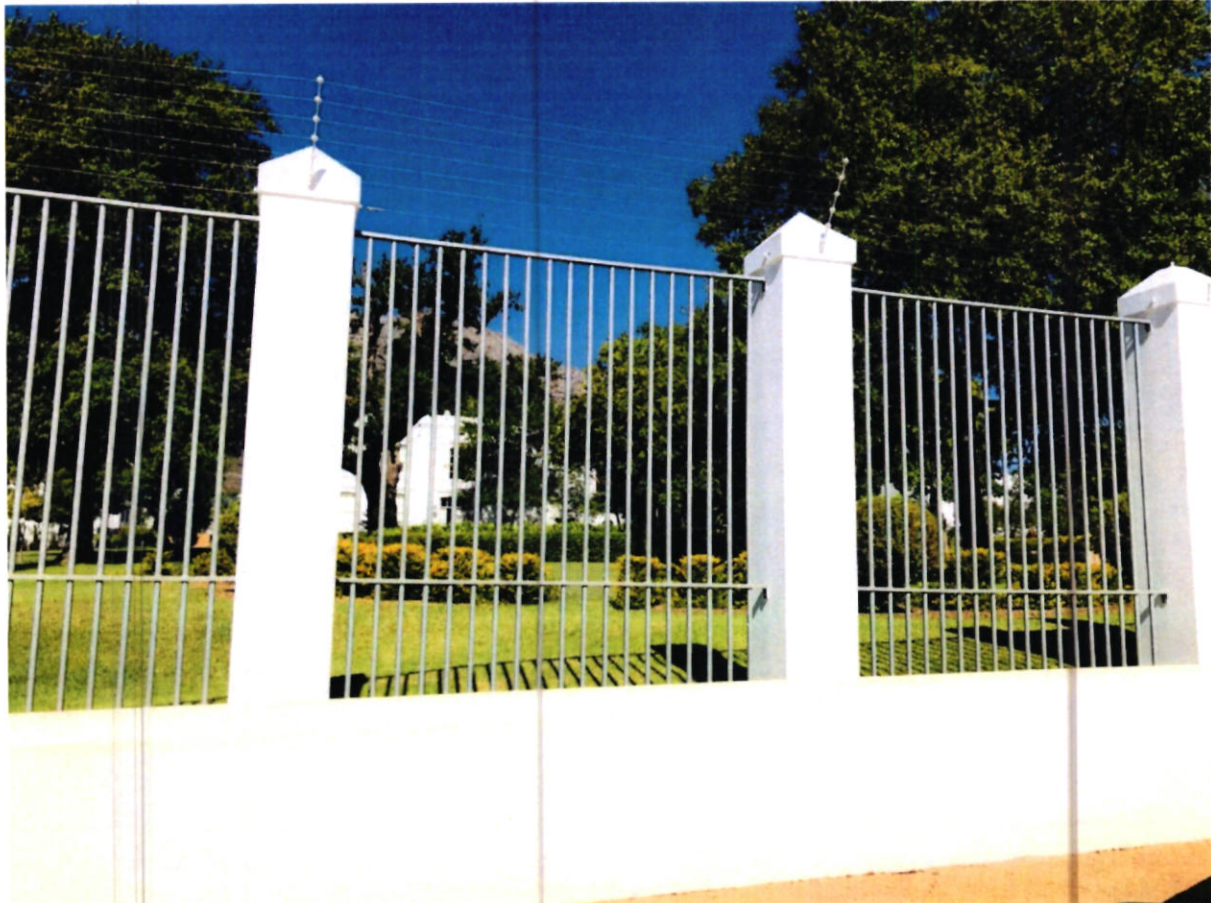
Figure 4: The enclosed and lawned farm werf of Brandwacht farm
