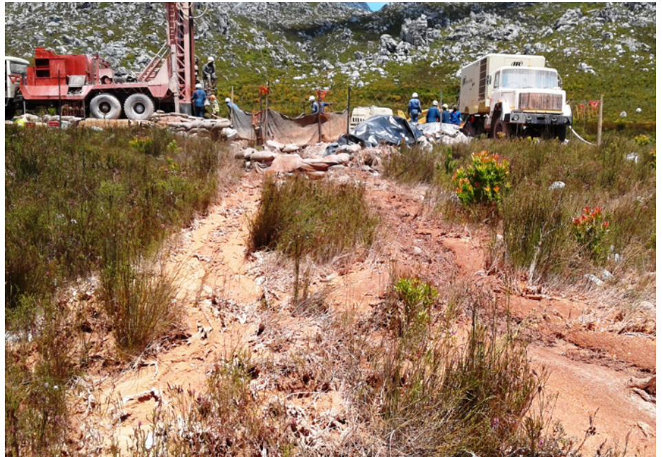
Fine sediments that escaped silt traps now coat the veld and adjacent streams.
