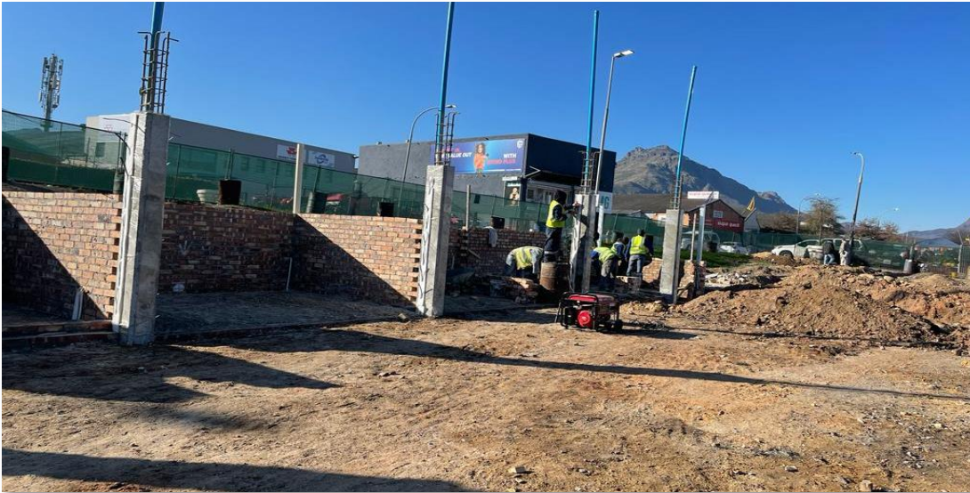
Figure 43: Construction of new taxi rank (Bird Street)
