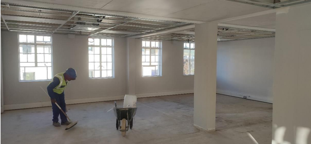
Figure 41: Upgrading of the NPK Building
