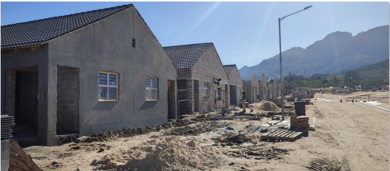
Figure 38: Ida's Valley Housing Development Project
