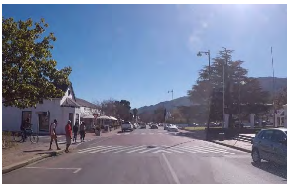
Figure 5: Franschhoek: Raised pedestrian crossing in CBD
