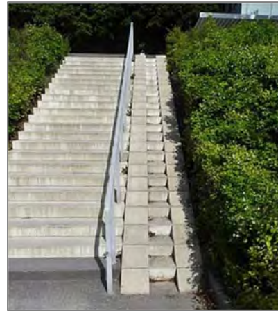
Figure 70: Proposed staircases with wheeling ramp to formalise access at locations of a steep slope gradient
